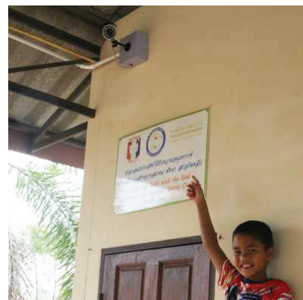
CCTV kamera ved Father Ray Childrens Village.
